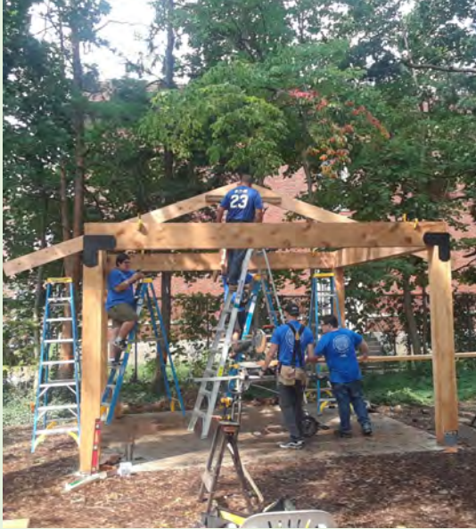
Photo 4: Pavilion structure to date
